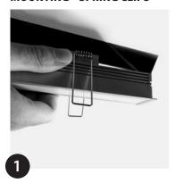
Cut 24-28 mm (0.94-1.10") wide slot to required length. Bring through power feed and make connection to LINI-R XL.
